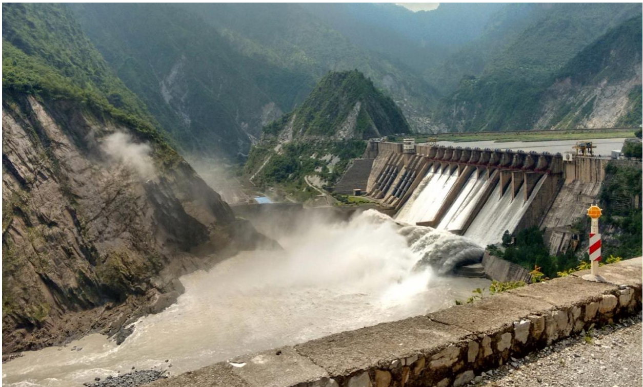
View of Salal Dam from Jyotipuram-Salal Road| Source: NHPC Limited
