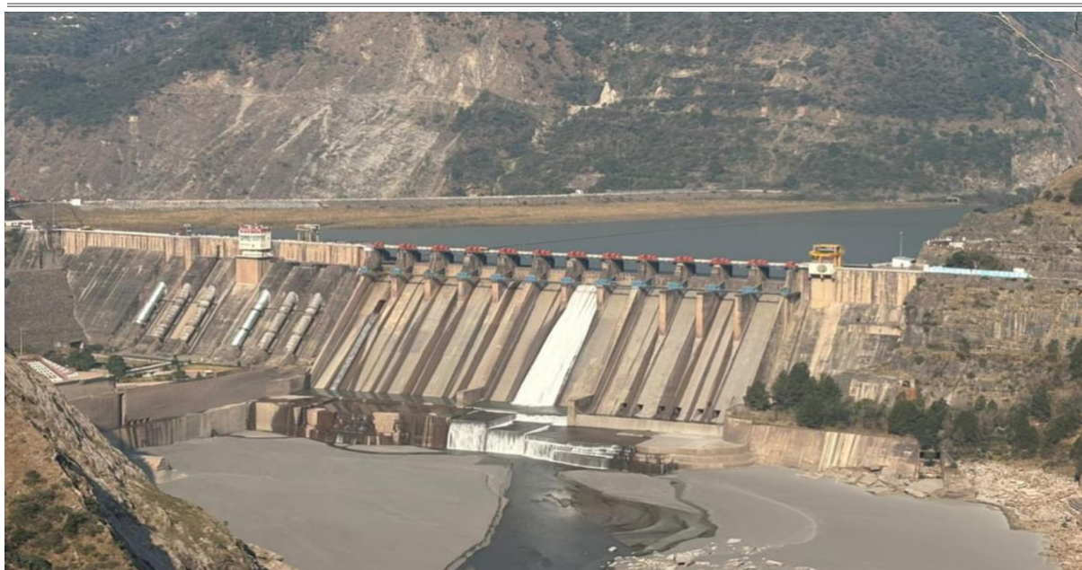
Figure 1: Salal Dam filled with sediments and vegetation but no water| Source: Pixaby
