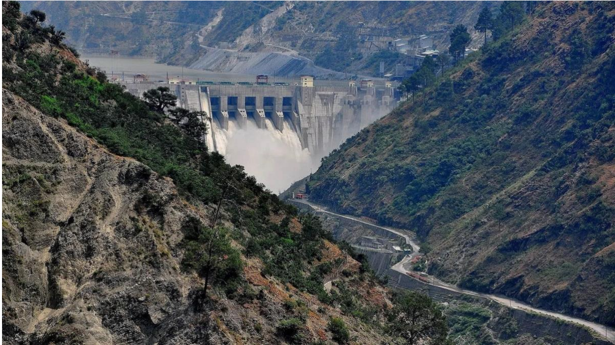
Ratle Hydroelectric Project | Source: Swarajyamag
